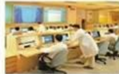
Control Center/Data Center
